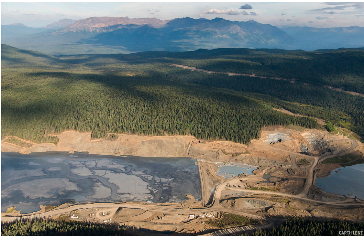
Red Chris mine tailings pond in northwest B.C.
