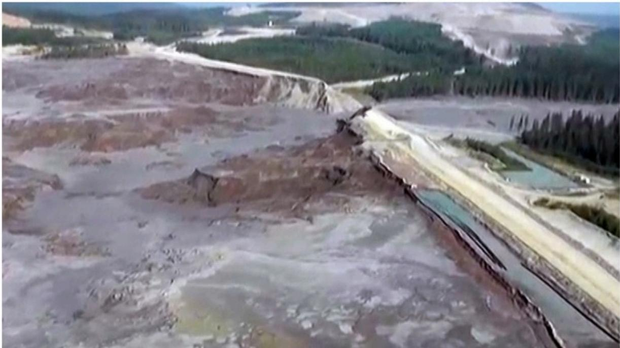
The breach of a tailings pond at the Mount Polley copper and gold mine in B.C. has released five million cubic metres of mining wastewater into local waterways. (Cariboo Regional District)
