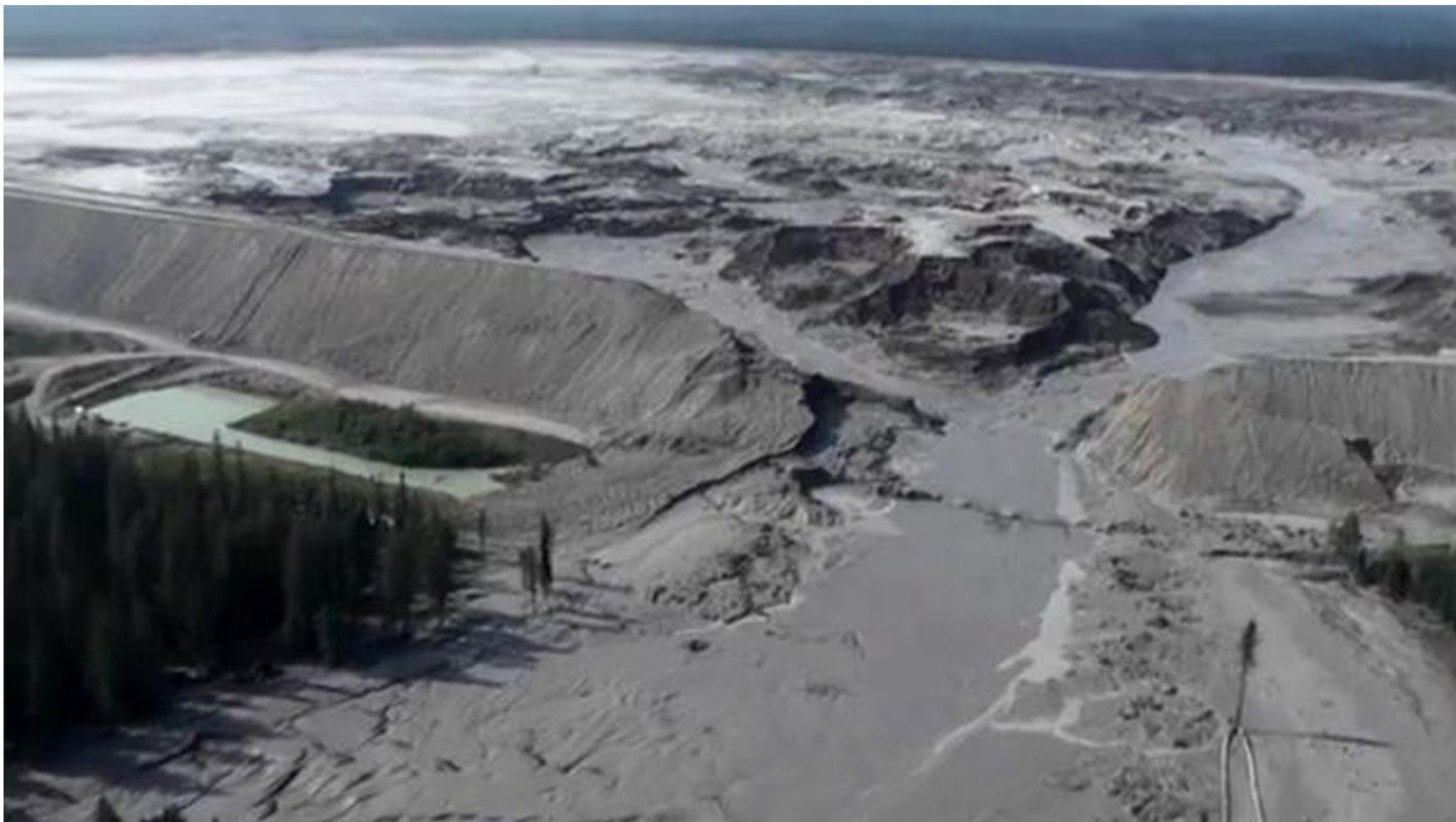
**A massive tailings pond breach at the Mt. Polley mine in 2014 spilled 24 million cubic meters of mine waste into a British Columbia watershed. (Photo credit: Canadian Ministry of the Environment)**
