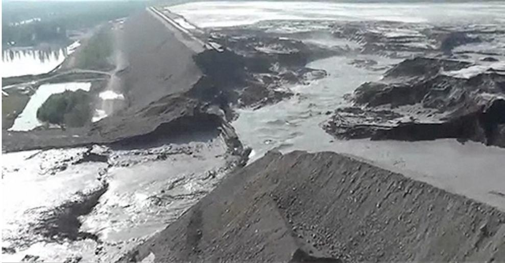
*Photo from Video of Mount Polley Tailings Storage Facility Breach*
